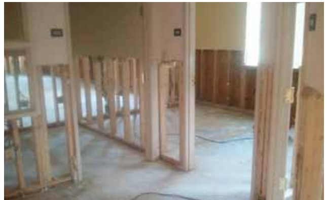
Gutted and ready for Drywall.
